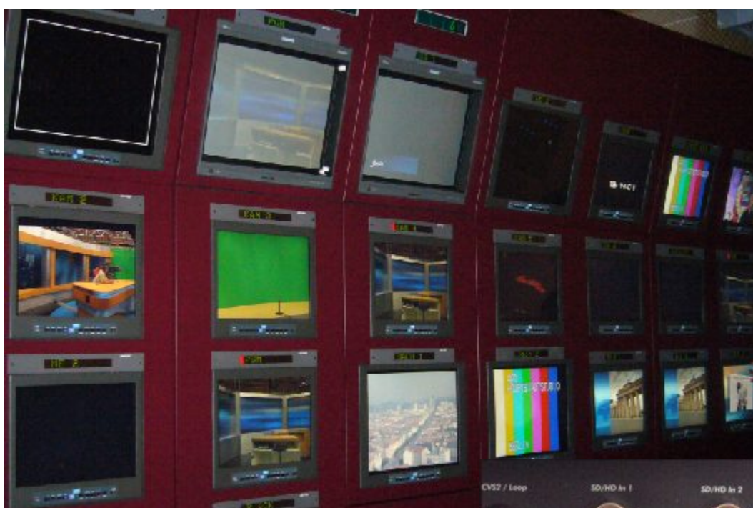
Customized Monitor Wall built with GREY OWL FLM 115 and FLM 120
